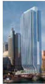
150 NORTH RIVERSIDE PLAZA 1.3M RSF
